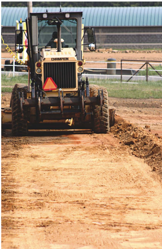
Finally at work on a multi-field sports complex in Heber Springs, Ark., this Champion motor grader operated by Cox Construction leaves behind a smooth grade, thanks to 3D machine control.
