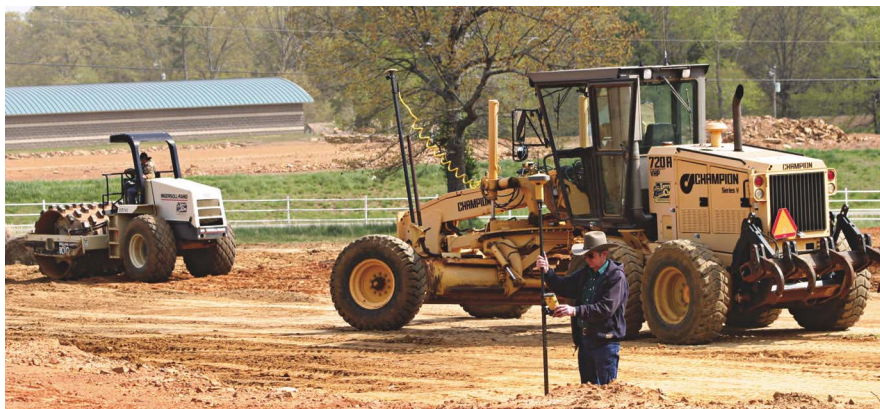
The land in Heber Springs, Ark., on which a multi-field sports complex is being built naturally has numerous slope changes. Here, earthmoving contractor Larry Cox stands on a low point, checking grade with his satellite receiver rover.
